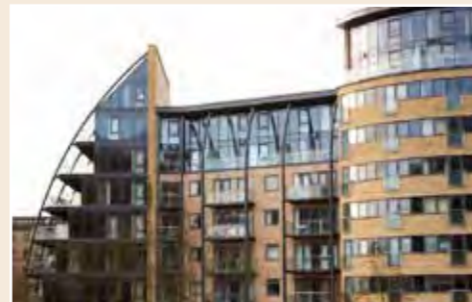
D Victoria Mills, Shipley was originally owned by the Jerome family who came from Limerick, Ireland, after being driven out during the 1904 antisemitic pogrom. The five acre site has recently been developed into approximately 400 residential apartments, within both new and converted buildings. The mill complex features three listed buildings, including a chimney, and the development has won various design awards. (Adapted from www.guardian.co.uk and www.newmason.co.uk )
