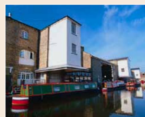
E The first section of this long range of Grade II Listed wool warehouses in Shipley was built in 1874. This building is situated at the eastern end of the range and is slightly taller and set further back from the canal than the others. A timber clad covered loading area extends over the canal. This feature would have helped to keep goods dry as they were unloaded. Although there are two later phases of construction, this group of warehouses retains a strongly consistent appearance including further covered loading areas. The warehouses were renovated in 1995 and their current uses include a restaurant and gym. (Adapted from www.bradford.gov.uk )
