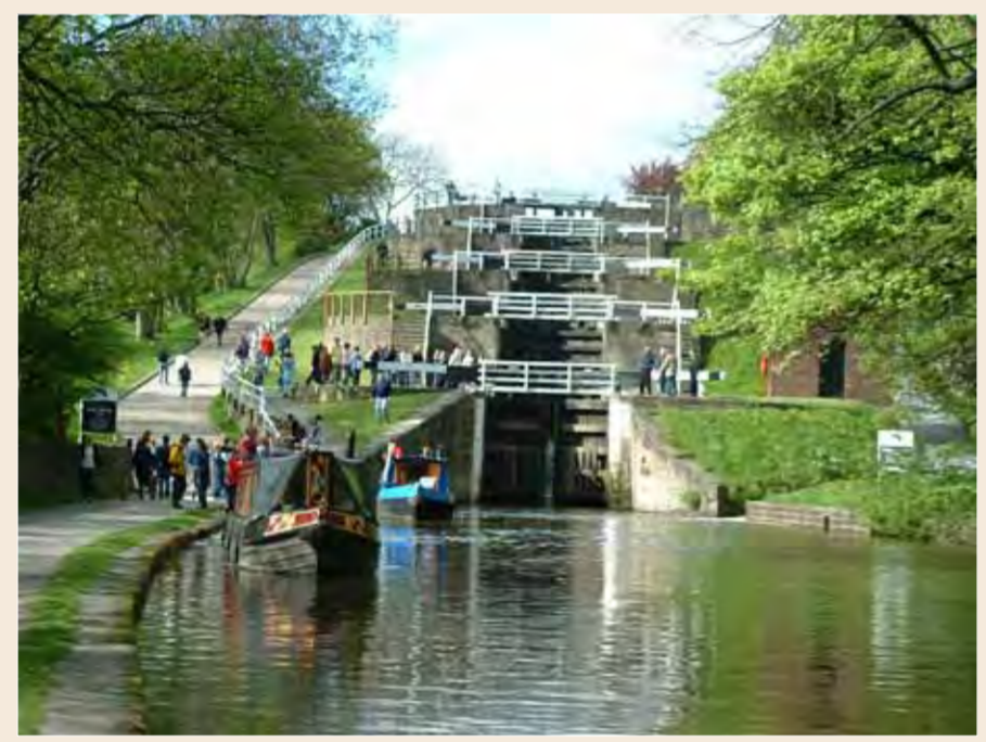
B Bingley Five Rise Locks are a Grade I listed structure and generally considered to be one of the finest feats of canal engineering in the country. Built c.1774 to the designs of engineer John Longbotham, the locks comprise of five locks in a stairway series that is preserved in a virtually unaltered condition since they were built and still in use to this day. The locks raise the level of the canal by 60ft and each lock holds 80,000-90,000 gallons of water. (Adapted from www.bradford.gov.uk )
